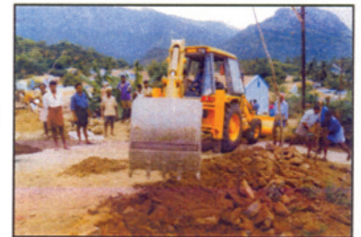
Improvement of road in the village (Foot path)
