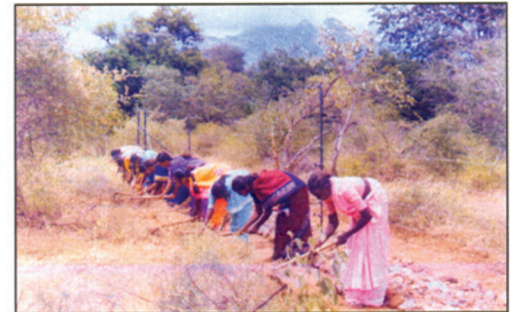
Members of WSHG involved in managing control plot solar power fence
