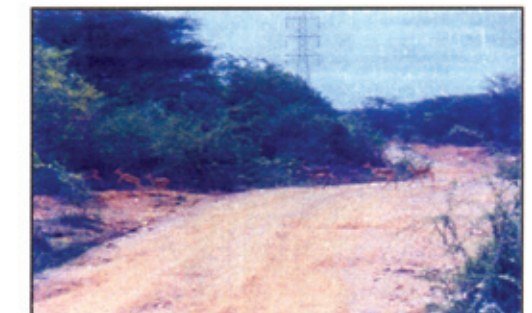
Establishment of road in elephant corridors
