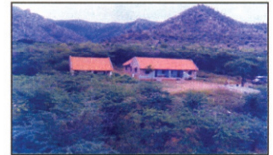
A renovated anti-poaching camp was established in Mangalapatti (Nilgiris North Forest Division)
