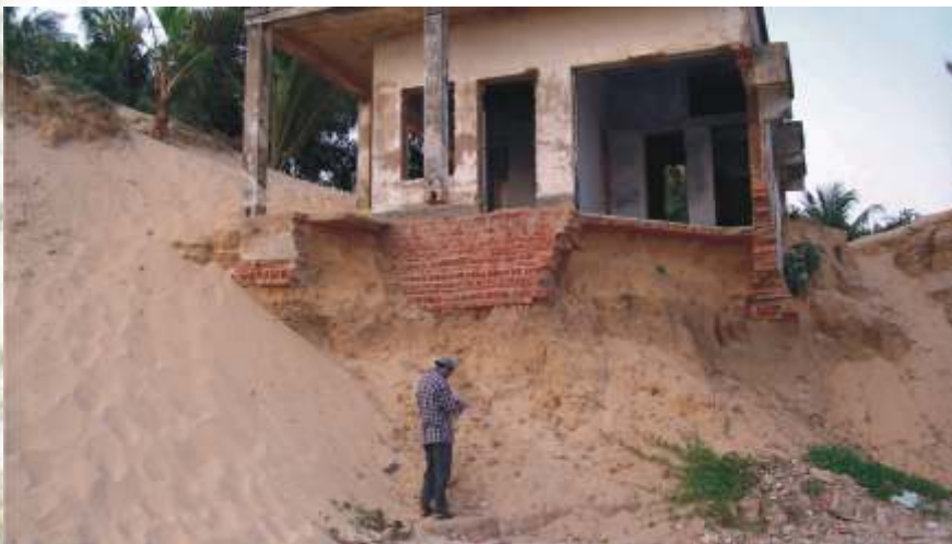
Fig. 8: The abandoned house of the Barrister Colony, Front on Digha Coast no longer exists
