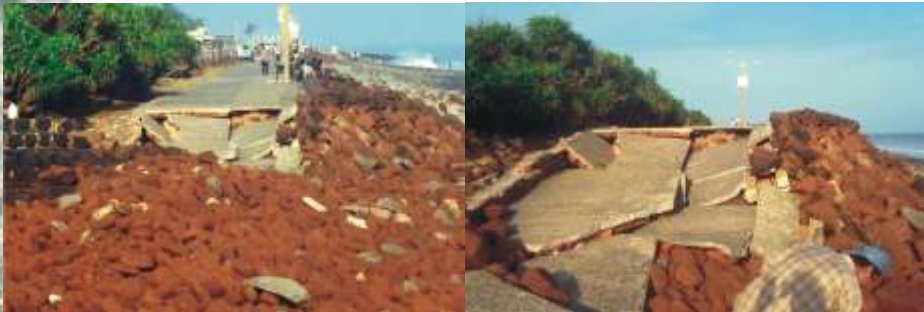
Fig. 12: Damaged parts of the Sea Wall after tidal surge
