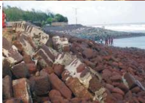
Fig. 12: Damaged parts of the Sea Wall after tidal surge
