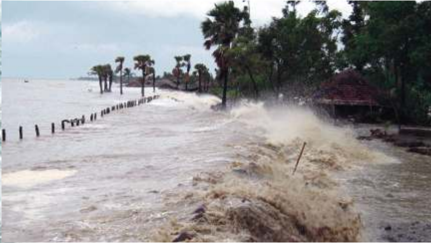
Fig. 14: Overtopping of Earthen embankment by a storm surge in Mousuni Island, Sundarban
